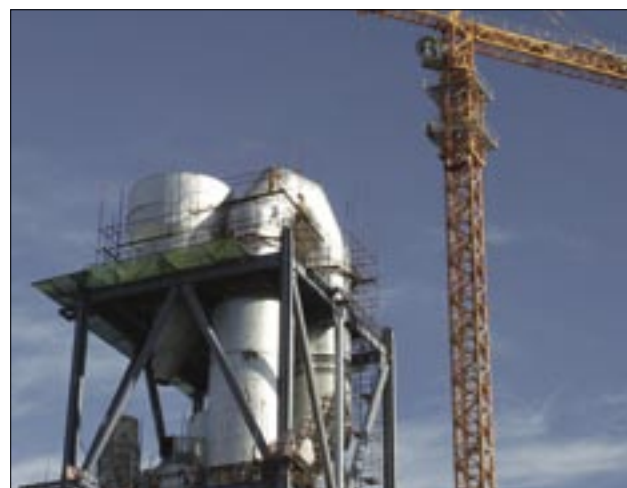
View of the pre-calciner tower under construction
