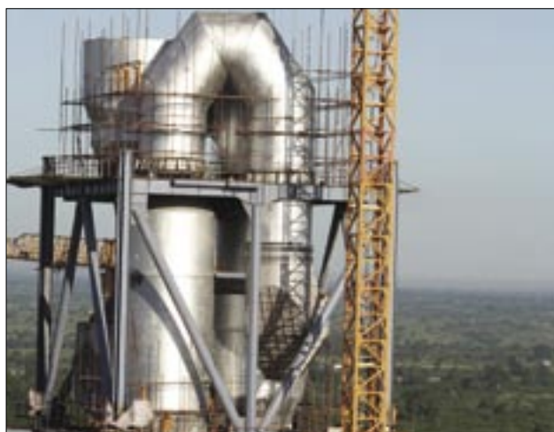
The 5-stage pre-calciner tower under construction
